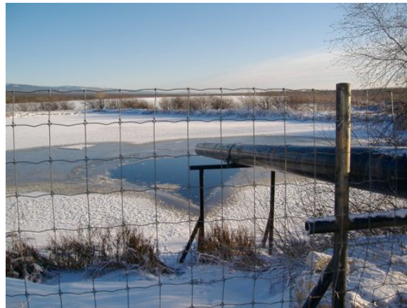
Norman Wells Sewage Lagoon
