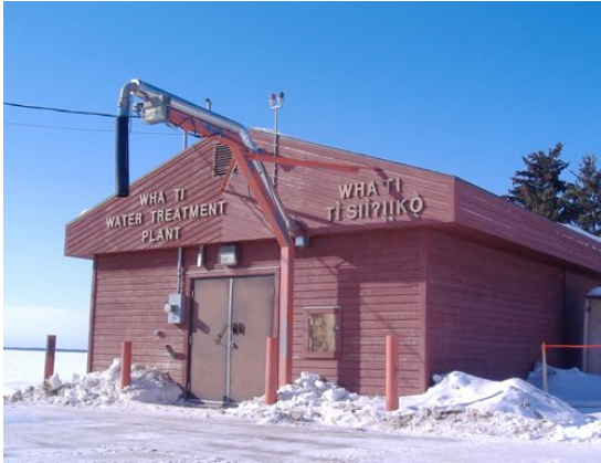
Wha ti water treatment plant
