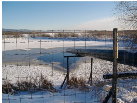
Norman Wells Sewage Lagoon
