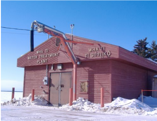
Wha ti water treatment plant
