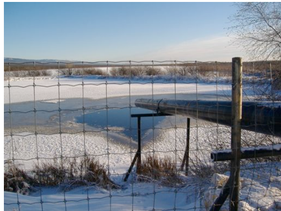
Norman Wells Sewage Lagoon
